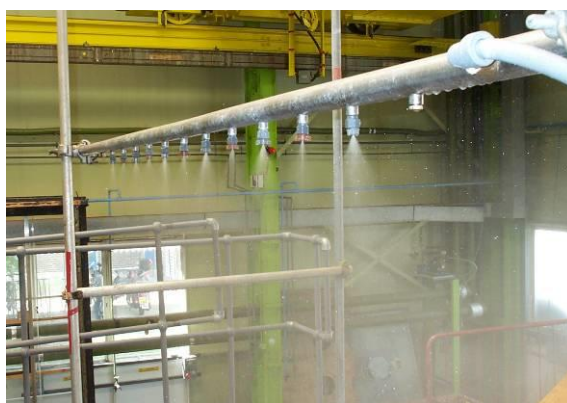
Figure B4 Top spray bar
