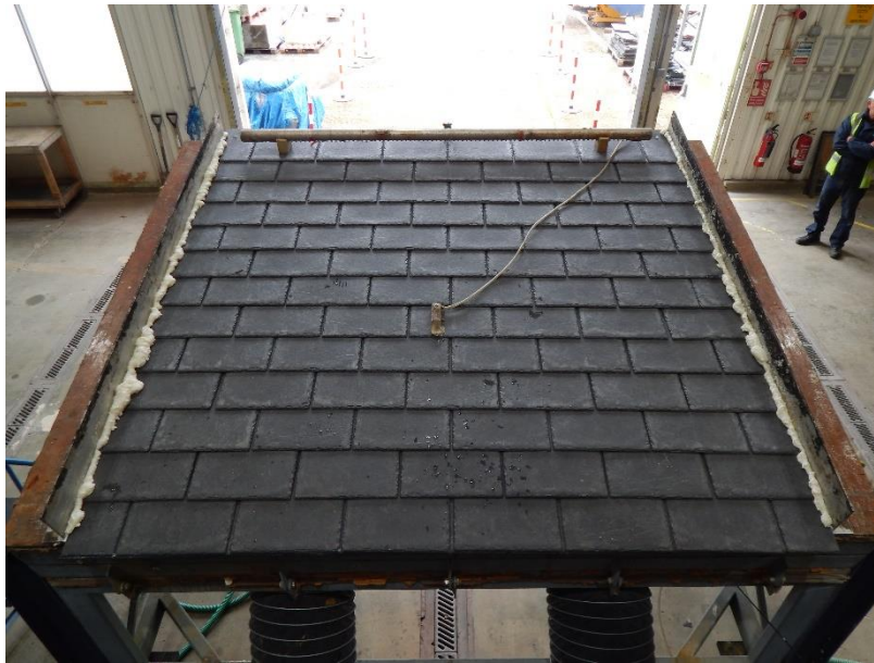
Figure 1. Installation of the Tapco Classic Slate on the BRE rig.
