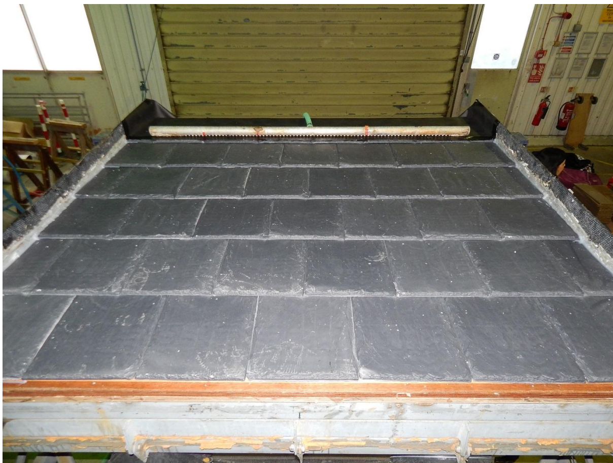
Figure 1 View of the Bellaforte Slate installed on the BRE test rig.
